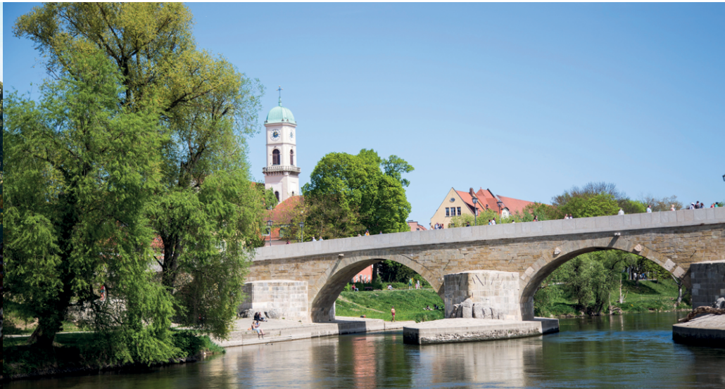
View of the stone bridge, Regensburg, Germany
